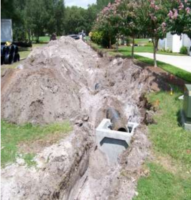
Figure 1-- Purple Finch Inlet box w/15" CPP under swale
